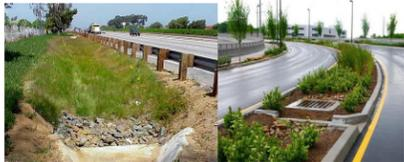
Figure 3: Vegetative stormwater control measures along roadways.
